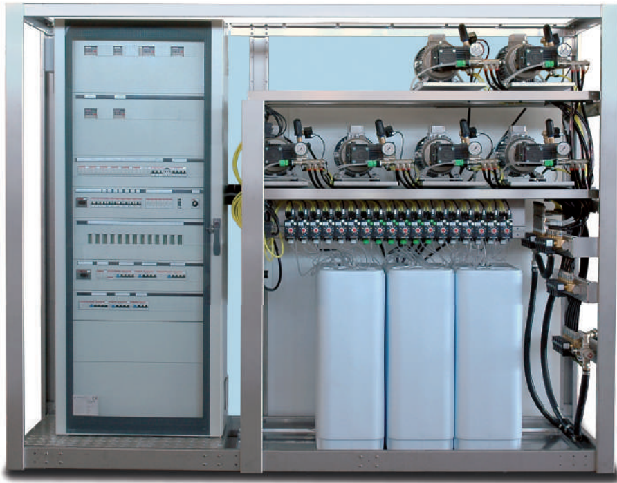
Aqua Rack: Telaio pompe e quadro elettrico Aqua Rack: Frame for high pressure pump and electric panel
